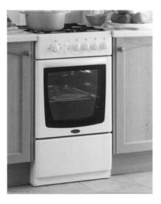
Unfortunate visual result of fixing a freestanding cooker in with standard cabinets by breaking the plinth line
